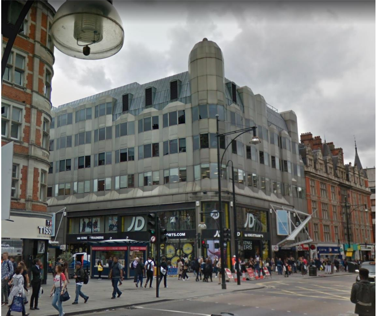
Oxford Street/Davies Street junction
